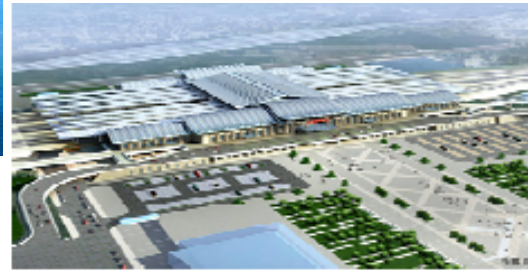
High-speed railway station
