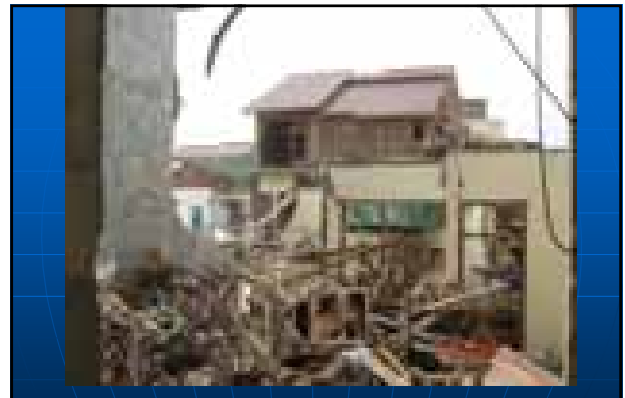
050128-100. Area of heavy destruction in the northern part of Banda Aceh, Sumatra, Indonesia
