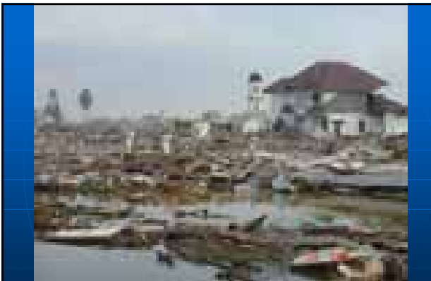
050128-071. At the limit of area of complete destruction in the northern part of Banda Aceh, Sumatra, Indonesia
